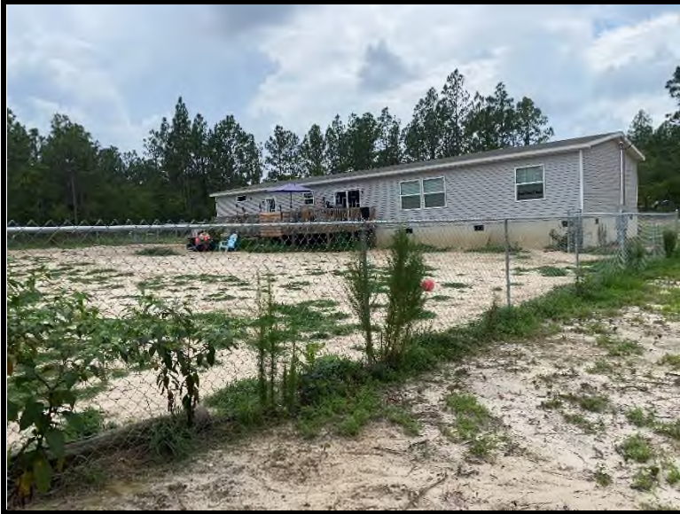
1 View of the residential structure located on the Property.
